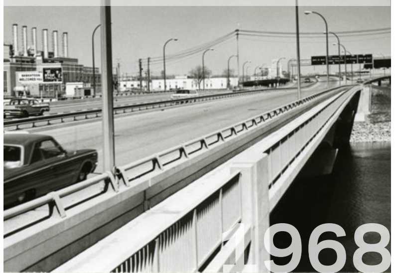
2. IDYLWYLD DRIVE BRIDGE
