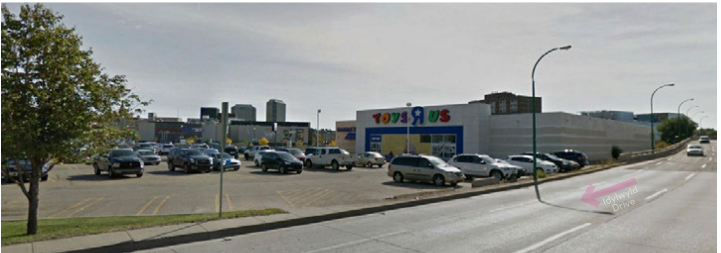
Figure 5.24: Block 2 Conditions Along Idylwyld Drive
