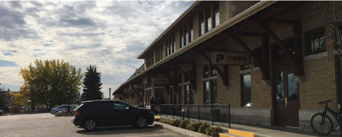
Figure 5.64: Block 9 Conditions Along Idylwyld Drive
