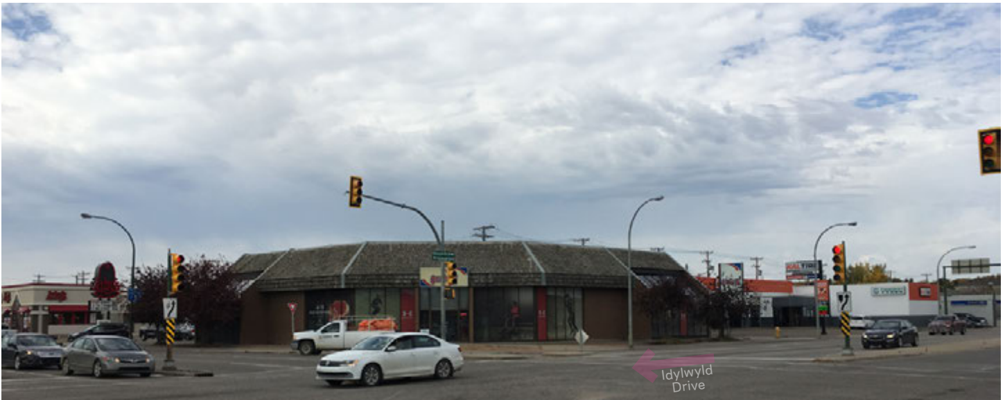
Figure 5.48: Block 6 Conditions Along Idylwyld Drive
