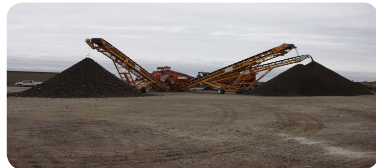
City of Saskatoon Nicholson Yard Material Handling site.
