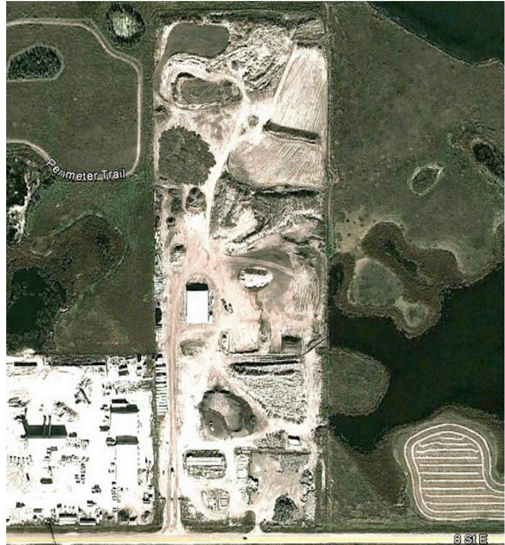
Aerial view of the City of Saskatoon Nicholson Yard Material Handling site.
