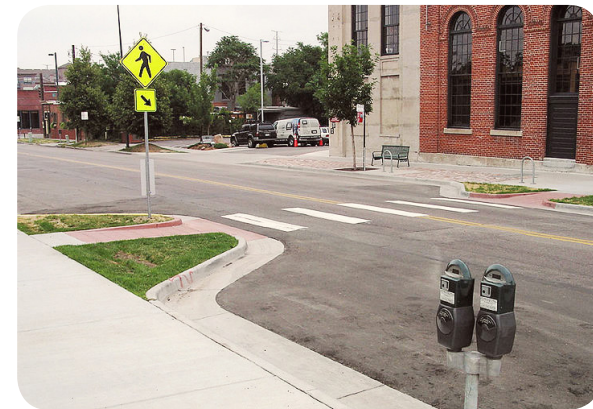
Traffic calming measures in the Brighton NCP: Curb bumpouts.
