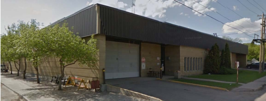
Parcel E – 1973 Building: Can be reused with strengthening of roof trusses.
