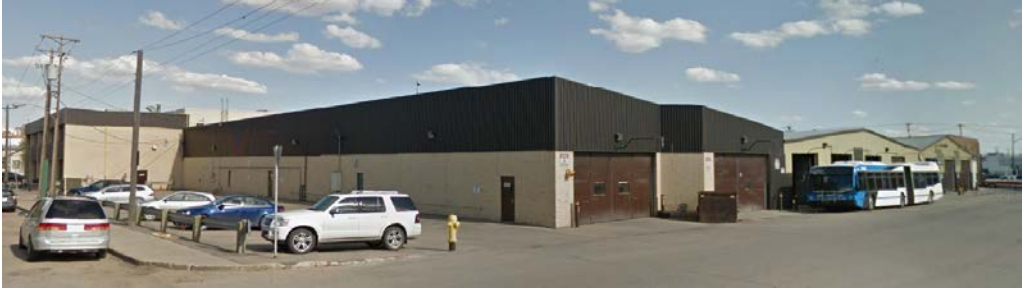
South Buildings: Demolition is most viable option.
