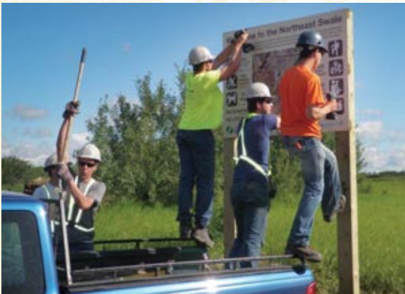
Top: River Landing Phase 2.
