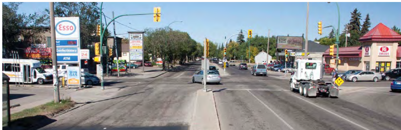
Figure 2.44 - Idylwyld Drive at 33 rd Street (looking north)
