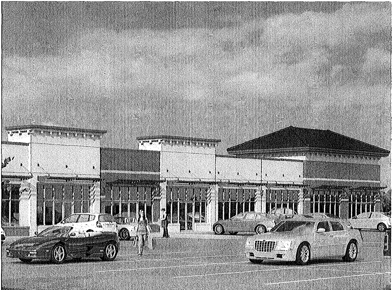
Stonegate Centre - 303 Cope Lane
