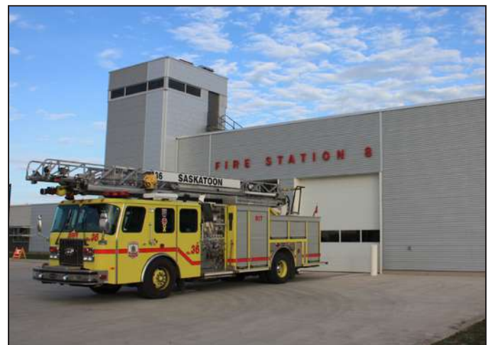
Fire Station #8 (Lakewood Suburban Centre)
