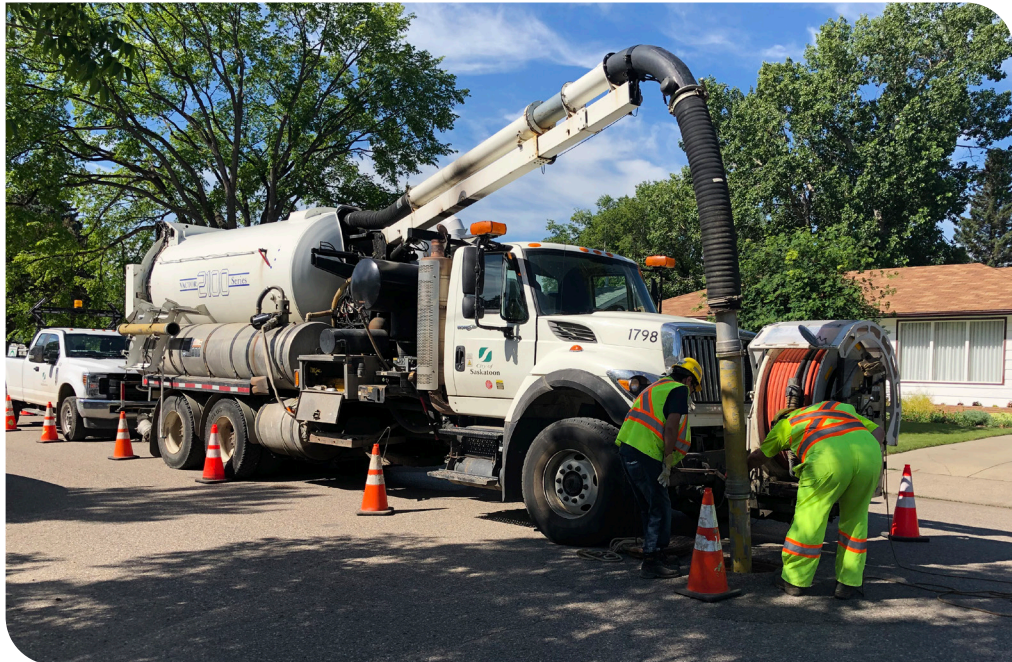
Sewer Flusher Vac Truck
