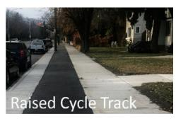
Raised Cycle Track: these facilities are located on the same level as the sidewalk, are typically separated from the sidewalk and are signed and marked for cyclist use only. There are 1.85 kilometers of raised cycle track in Saskatoon.
