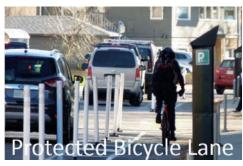
Protected Bicycle Lanes: these facilities are located on the street, buffered from traffic by a combination of space, curbing, planters, parked vehicles, and/ or delineator poles. This facility type was used for the temporary installation for the downtown protected bike lane demonstration project. There are over three kilometers of protected bike lanes in Saskatoon.
